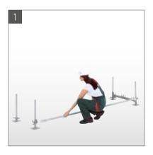
Set up adjustable base jacks, place lower diagonal fasteners, mounting guard rails (only in the diagonal field).
