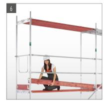
Assemble vertical frames and decks of the next level, then mount diagonal braces, guard rails and toe boards.
